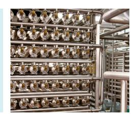
Nanofiltration (NF) sanitary spiral elements have been designed to separate monovalent ions from mixtures of monovalent and multivalent ions, while rejecting organics.
